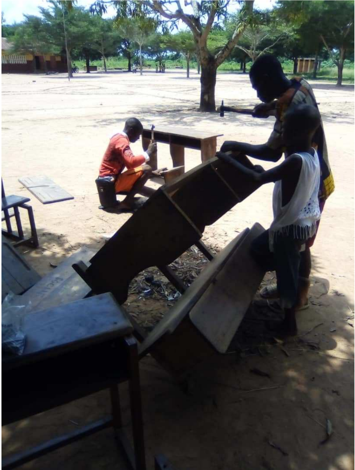
ONGED repairs spoiled desks at the school of Kpodaha
