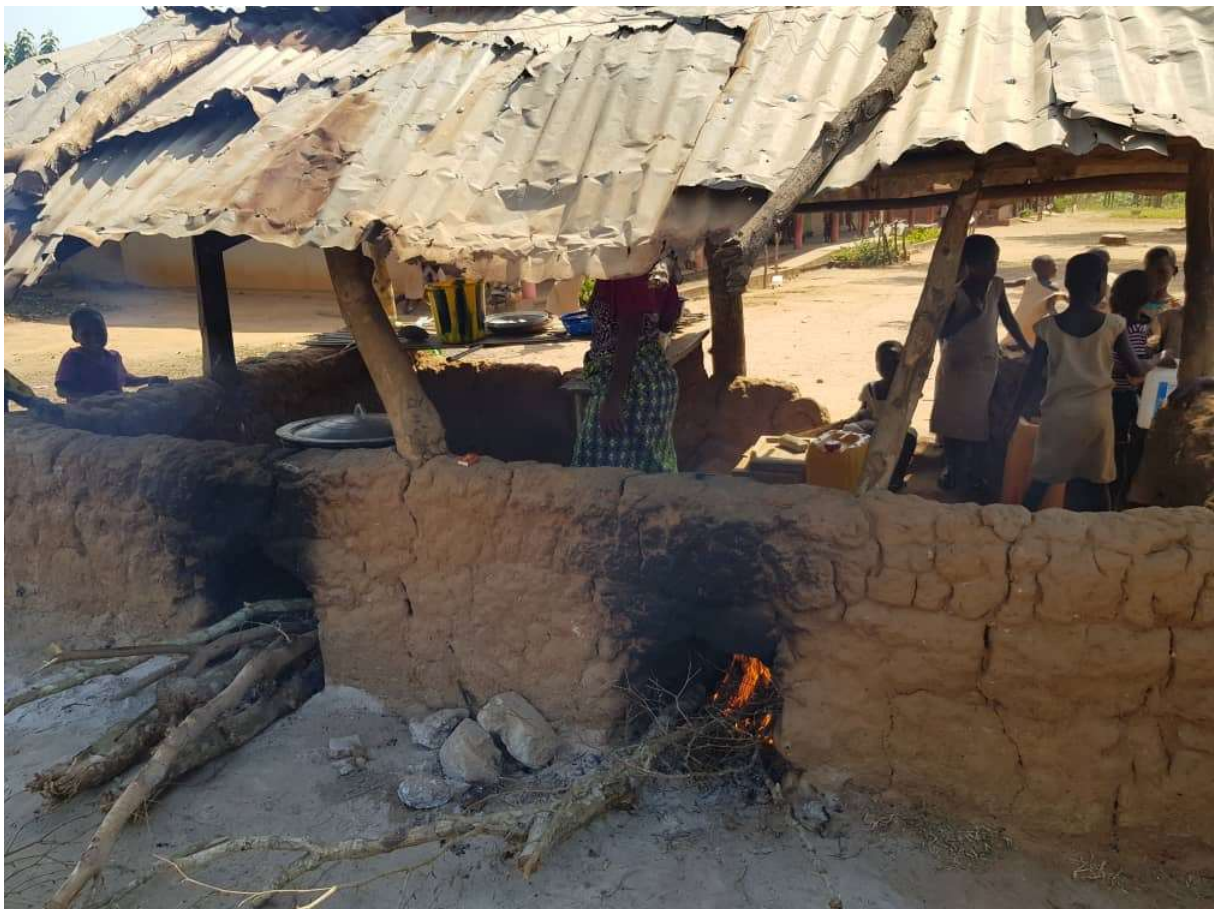
A kitchen that does not meet school canteen standards
