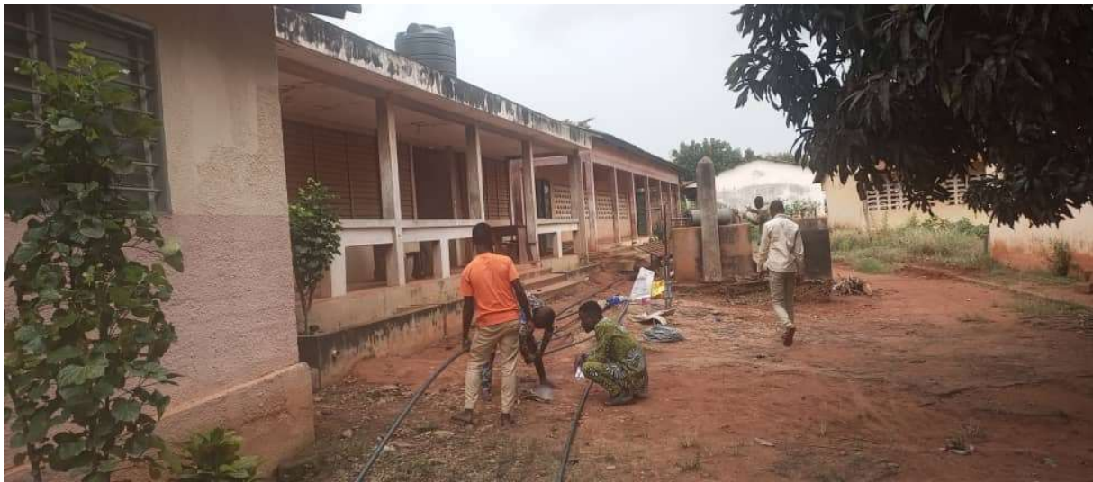
Technicians at work on the water tower
