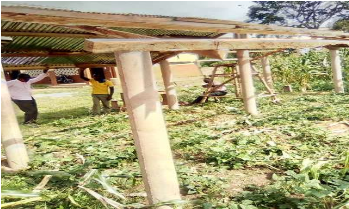
Kitchen under construction
