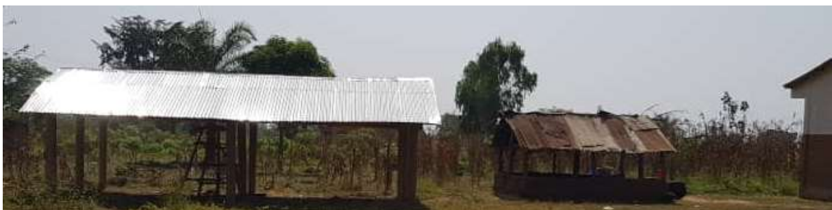
New kitchen built next to the old one
