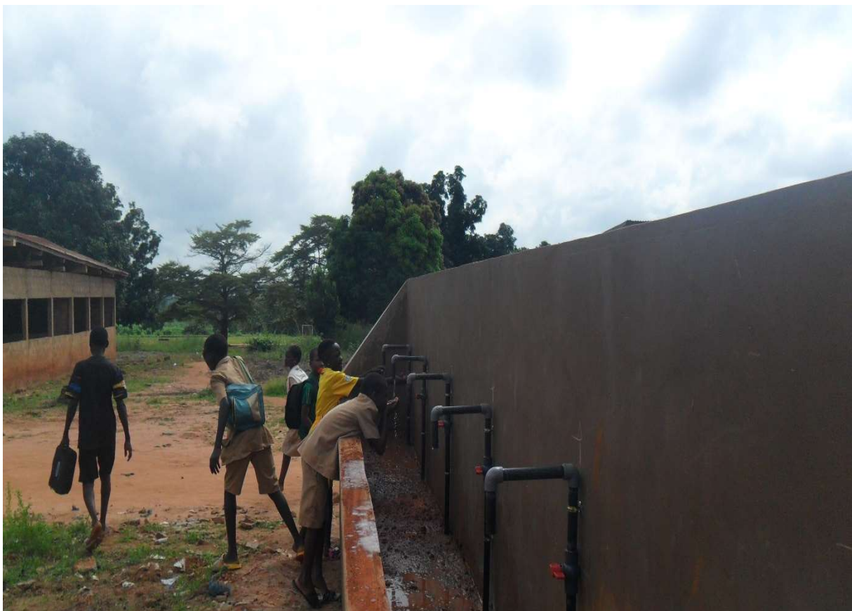
Students using water before the completion of the hand wash
